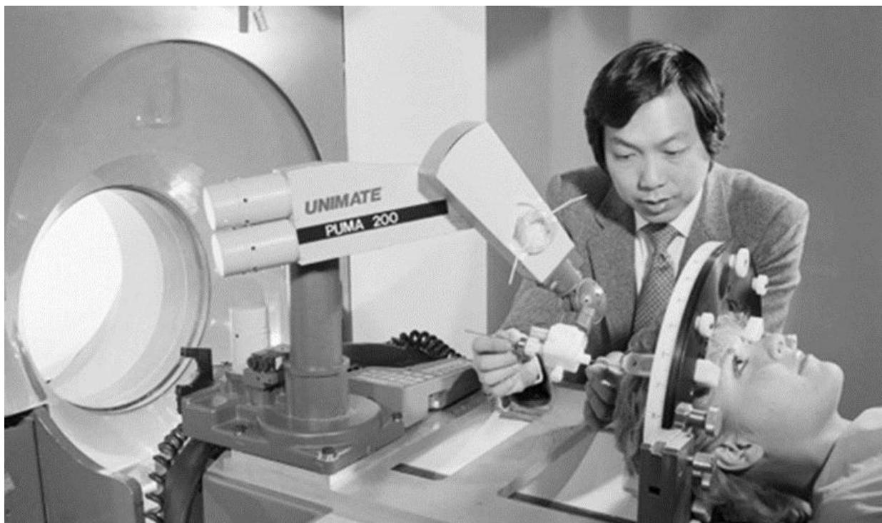
**Figure 73: Programmable Universal Machine for Assembly (PUMA® 200)**
